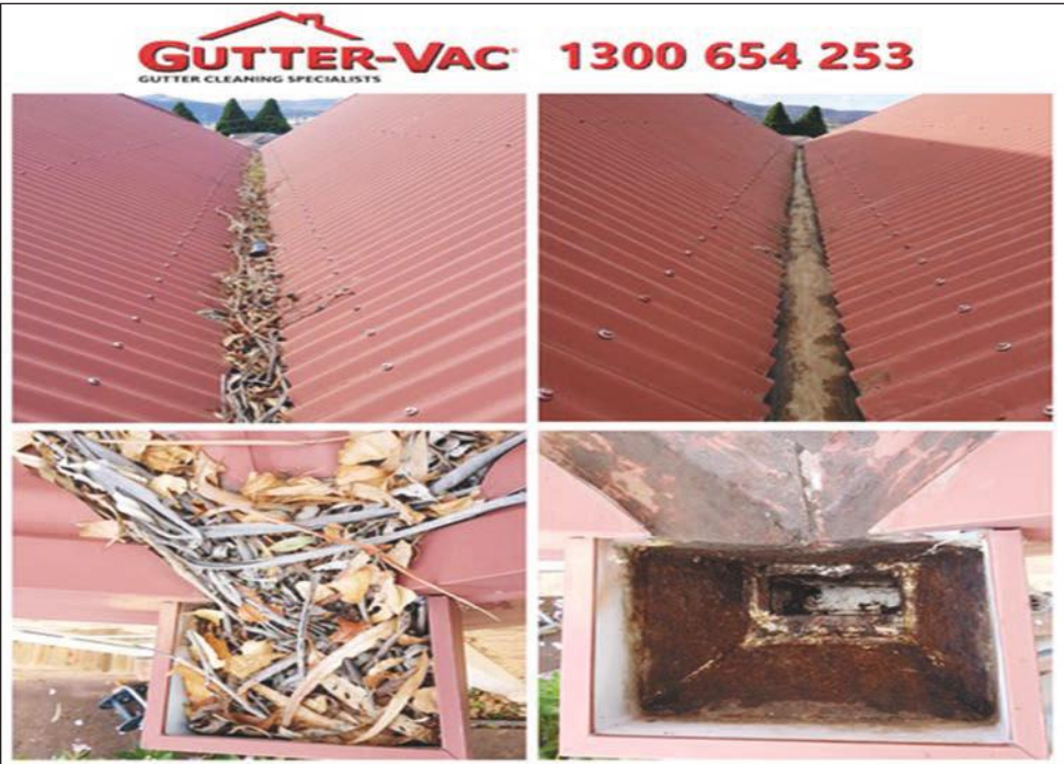
Debris in gutters act as kindling for embers (in the 'before' image on left). Gutter-Vac Southern Tasmania professionally removed the debris (shown in 'after' image on right). (PS)
