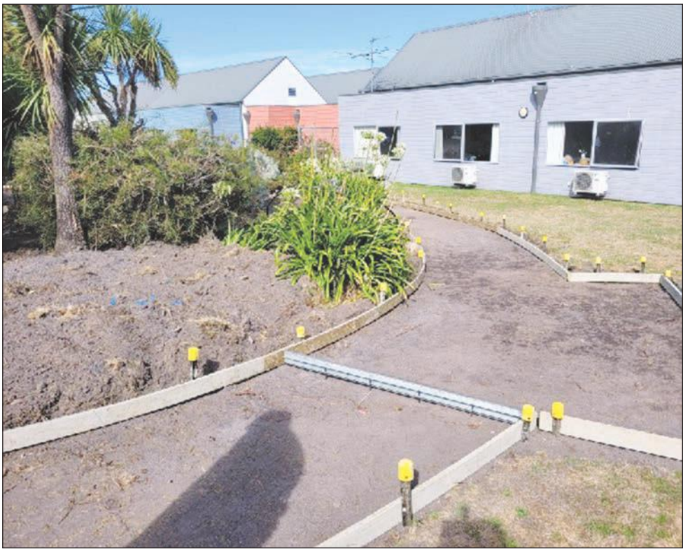
The area was a bit unloved and in need of some attention. The garden has been cleared of a lot of old trees and rubbish, and machines came in to dig the pathways and set them up for the concrete pour. There are now pathways wide enough for wheelchairs and walkers throughout the garden. (PS)
