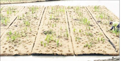
The floating wetlands being planted with carefully selected vegetation which will grow through the rafts and the water column creating a large treatment mat which is 300 per cent more efficient than a standard wetland treatment system. (PS)
